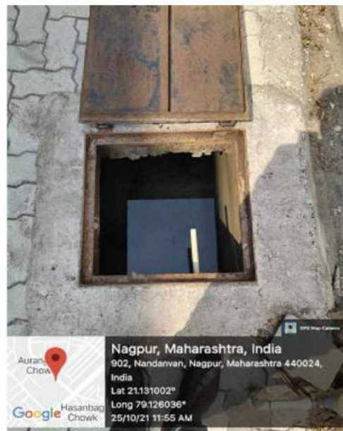
Tank constructed in college
