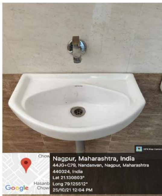
Taps to be replaced by faucets
