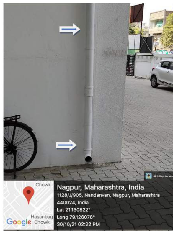
Rain Water Harvesting System under construction
